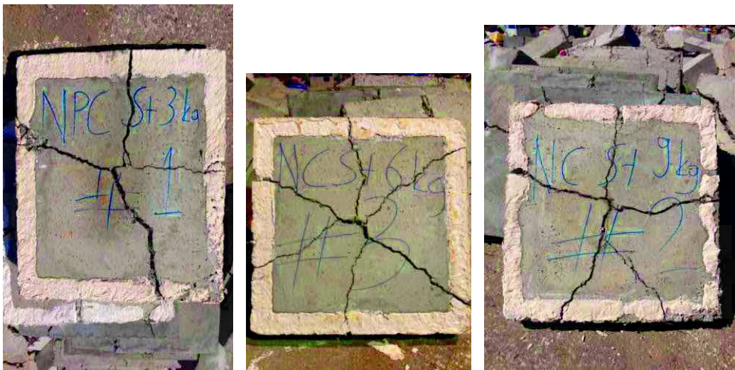
Fig. 5. Crack pattern for Normal Performance Concrete (NPC)
