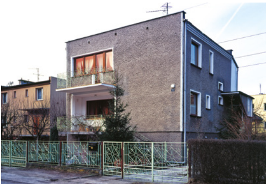
Before thermal modernisation
