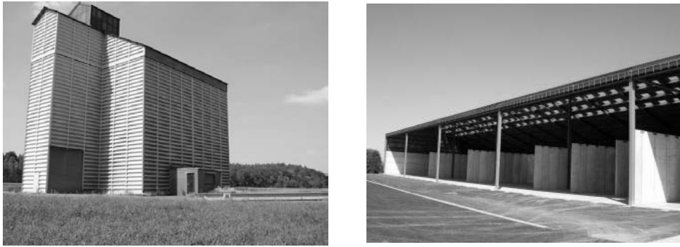
Figure 1 : Two main storage facilities in Wallonia : ACMB (left) and Silo Box (right)
