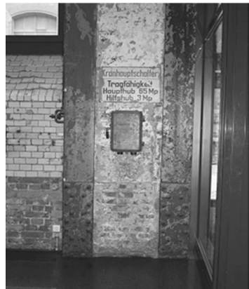
Photo 5. Functional details of the former power plant become decorative elements in the new space, September 2017 (Magdalena Abraham-Diefenbach)
