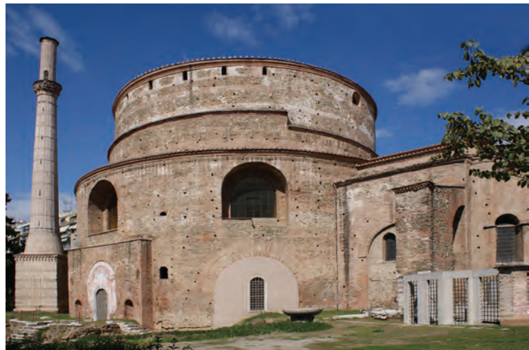
Fig. 5. Rotunda, view from the south, with Christian apsis, and the main entrance from the first stage of its construction (photo by R. Szlązak)
