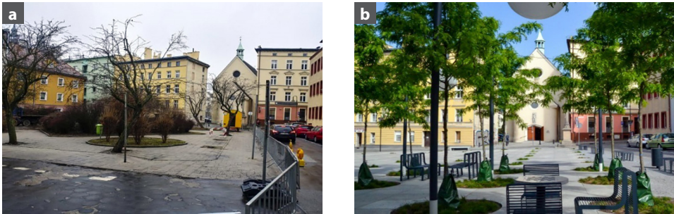
Fig. 6. Saint Sebastian Square: (a) before renovation, (b) after renovation
