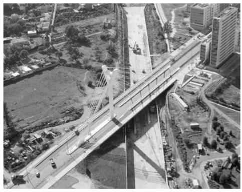
Fig. 15. The new bridge over the "Seco" (dry) river was also design in an attempt to benefit sustainable means of transportation: wide sidewalks, cycle path, only one lane per direction for cars Source: author collection
