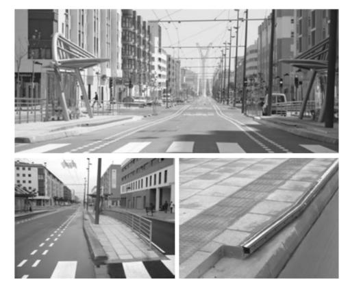
Fig. 7 and 8. In Castellón a particular concrete kerb was designed to help the guidance system align the vehicles to the stops Source: author collection
