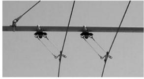
Fig. 10. The vertical elements were specifically designed for Castellón and hold the lighting system and the catenary Source: author collection
