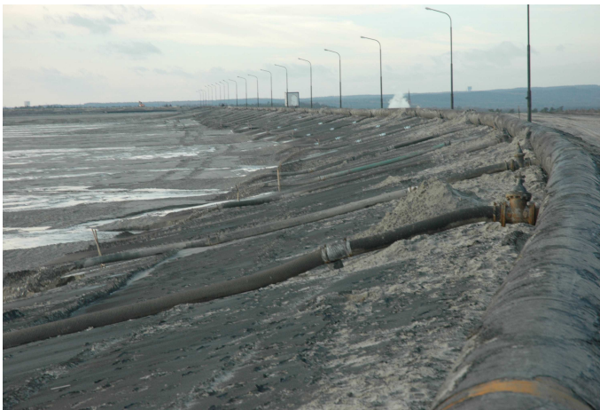
Fig. 1. Spigotting outlets in Żelazny Most tailings pond (KGHM Polska Miedź S.A., Poland)
