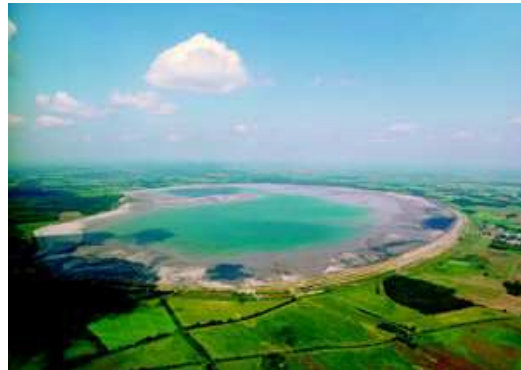
Fig. 6. Ring-Dike type of impoundment structure (left), tailings pond Želazný Most (right)
