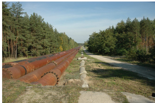
Fig. 11. Slurry transporting system between KGHM mines and Želazny Most tailings pond
