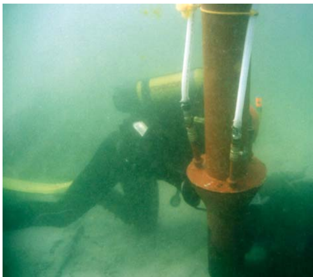
Fig. 17. A scuba diver clears away sand from the hull remains using a large airlift fed by two air compressors (photo by W. Ossowski).
