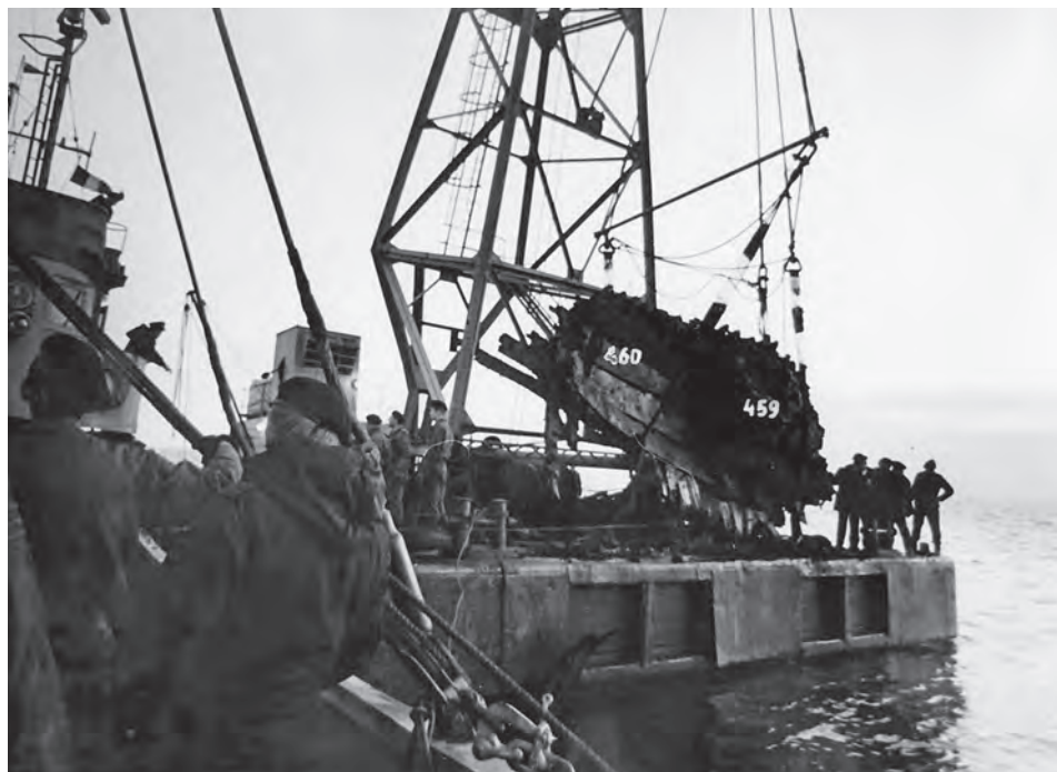
Fig. 23. The principal structural section of hull, complete with a concreted mass of cargo, salvaged by the Polish Navy on 17 October 1975 (photo by L. Nowicz).
