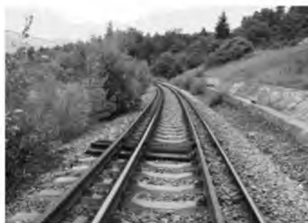
Figure 6. Double Railway System: European (normal, Romania) and ex-soviet (large; Ukraine) in the Romanian borderland
