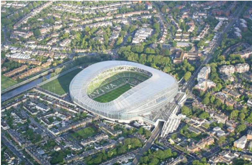
Fig. 1.3. Aviva Stadium in Dublin, Ireland [ www.avivastadium.ie ]
