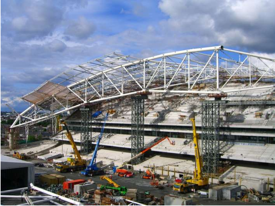
Fig. 2.11. Horseshoe truss construction process [www.grasshopper3d.com]
