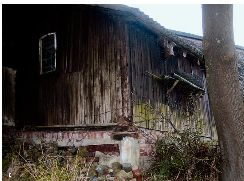
Fig. 3. Barns built with jaw bone supports. a) Whitby, Co. North Yorkshire, England, during demolition in 1930 (photo: Frank Sutcliffe, Whitby Museum; from Redman 2004:171); b) Bremen-Lesum, Lesumbroker Landstraße 111, during demolition in 1906 (photo: Focke-Museum Bremen, inv. no. B.477e); c) Bremen-Lesum, Niederbüren 2, barn with jaw bone segments in foundation (photo: Susanne Henßen 2009)
