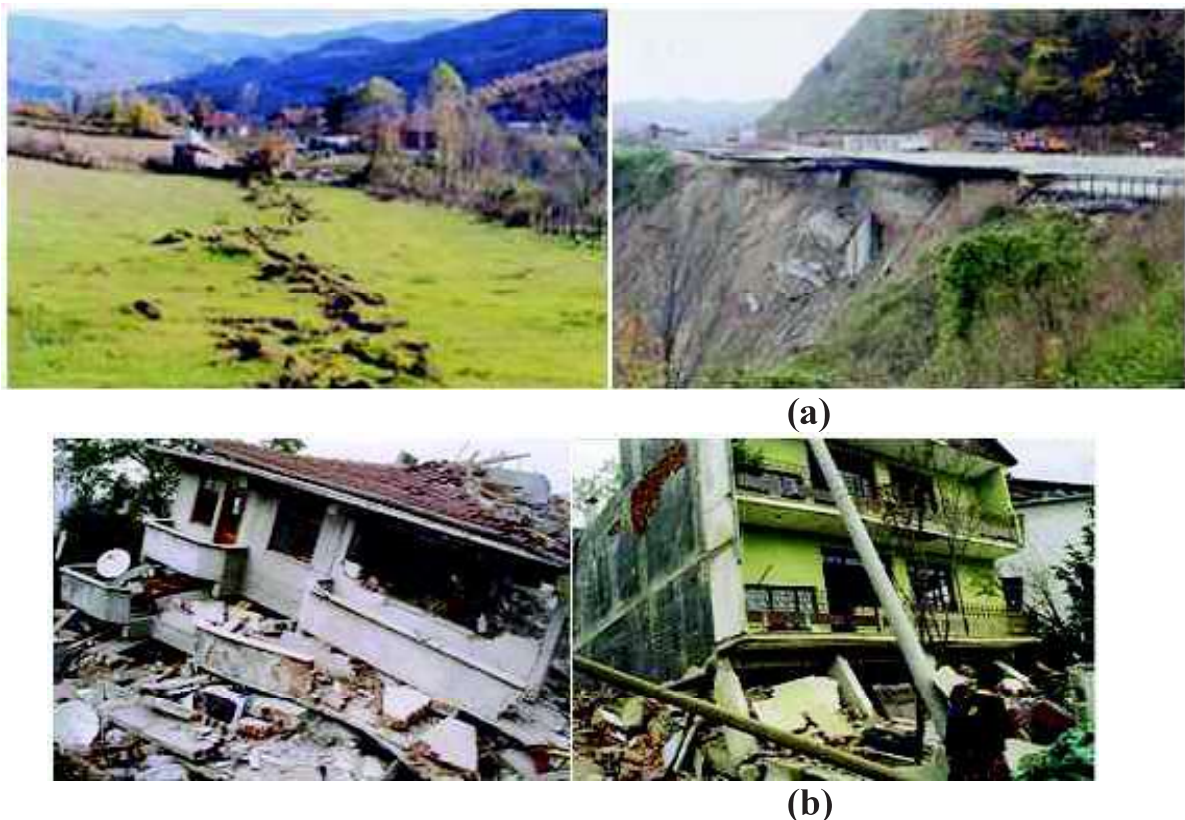
Fig. 13. Buildings was damaged, and evacuated after the 12 November 1999 Duzce EQ
