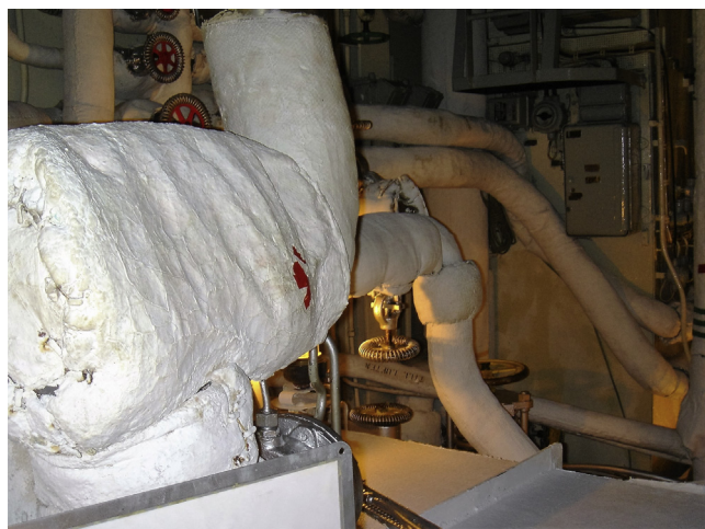
Fig. 1. Asbestos heat insulation in a retired Swedish submarine (photo by Adam Pawelczyk).
