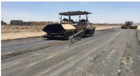
Fig. 9. Paving finisher waiting the asphalt trucks
