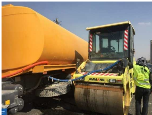
Fig. 11. Double drum rollers filling with water
