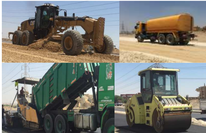
Fig. 7. Road project machines
