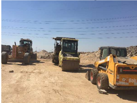
Fig. 8. Waiting for inspecting the finished activity
