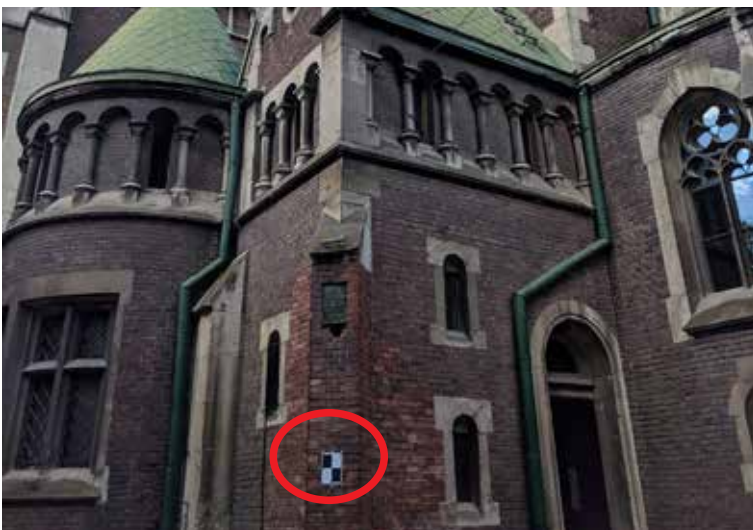
Figure 5. Picture of the visor mark on the building
