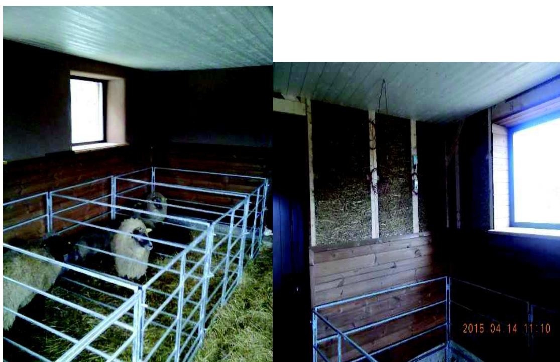
Fig. 1. Sheepfold made from wooden panel with straw filler and detectors, transmitters, controllers for temperature regime monitoring
