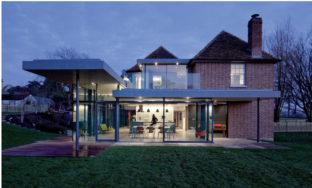
Figure 1 A crucial challenge facing lighting professionals today who design residential lighting schemes, is to provide LED lighting that is both visually safe and harmless to general health. Pic: Light.iQ
