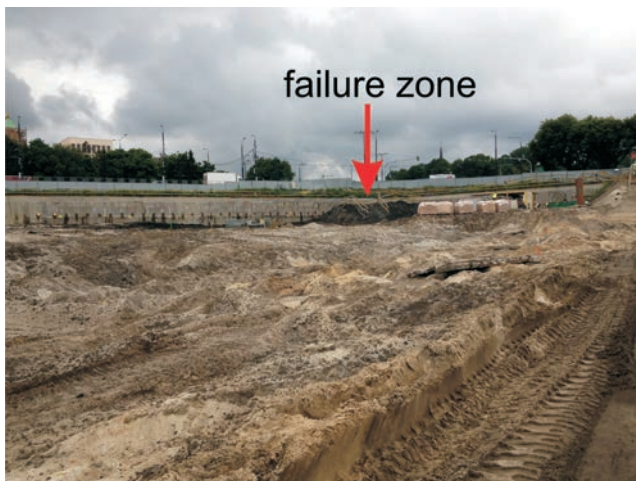
Fig. 1. View of the NW part of the foundation trench.
