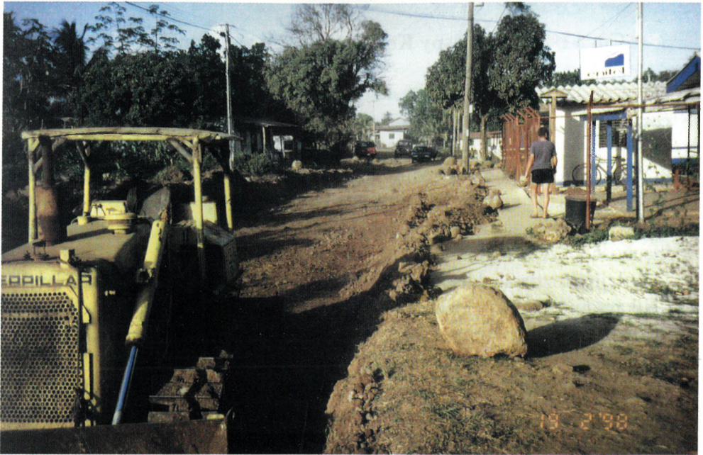
9. New „Enitel” telephone company and roadworks
