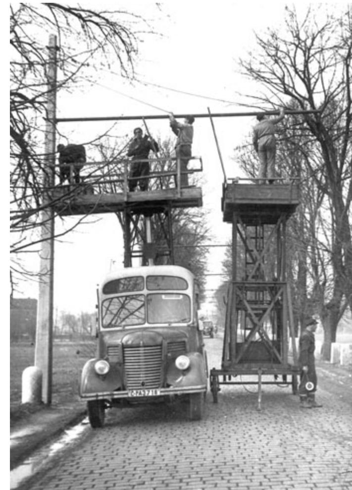
*Fig. 1. Construction of the first trolleybus line to Lázně Bohdaneč
