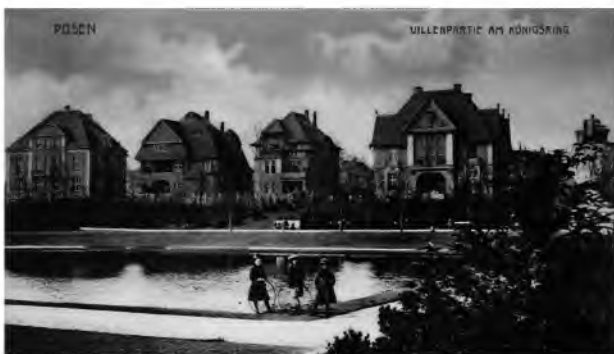
FIG. 4. Hygiene Institute of Posen (Poznan), around 1913 (left-most position), Source: Adam Mickiewicz University Library, Poznan, Poland
