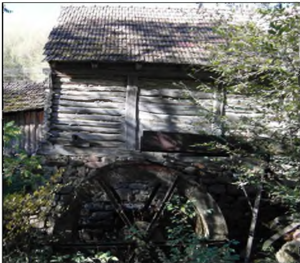
Fig. 8. Water mill from Vărciorog village
