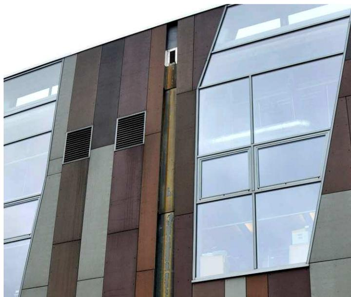
Rys. 2. Marks of the water flowing down the breaches in the facade (fot. G. Grzełiński)
